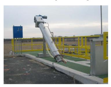
AquaTec screens are suitable for Municipal wastewater plant headworks or Industrial water screening. The photo at the right shows the typical "on-line" operation. "Shaftless" self-cleaning operation is nearly clog-proof. These low cost screens are easy to install and maintain.
